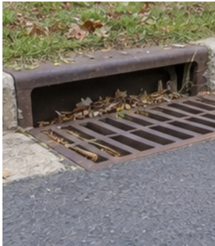
Photo 2: Catch basin at the curb.
