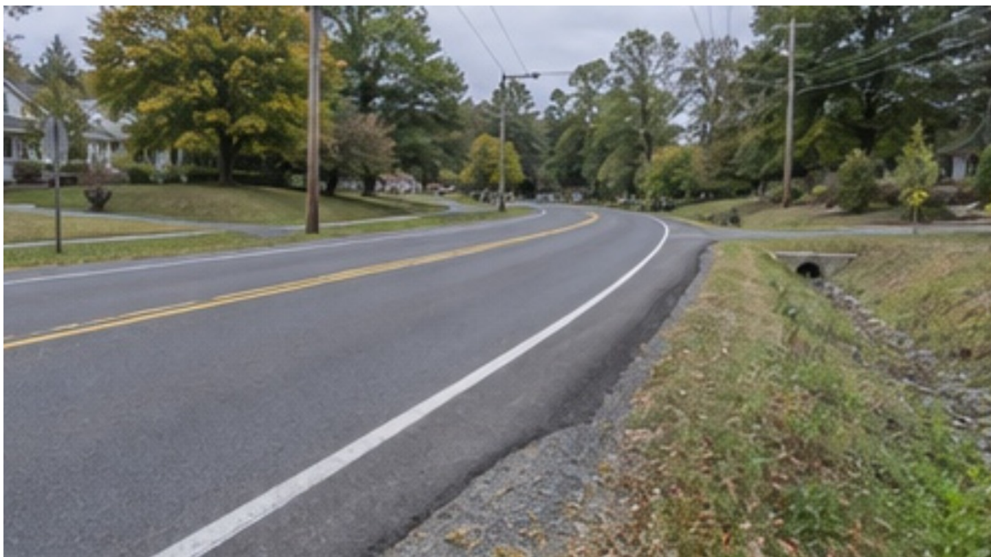
Photo 6: Roadway approach and roadside ditch.
