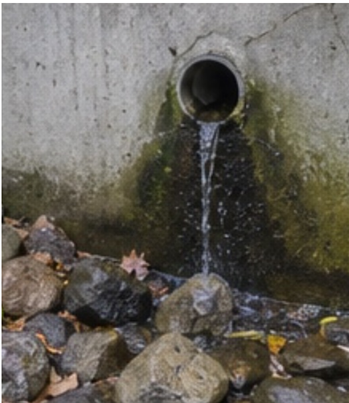
Photo 3: Retaining wall drainage outlet.
