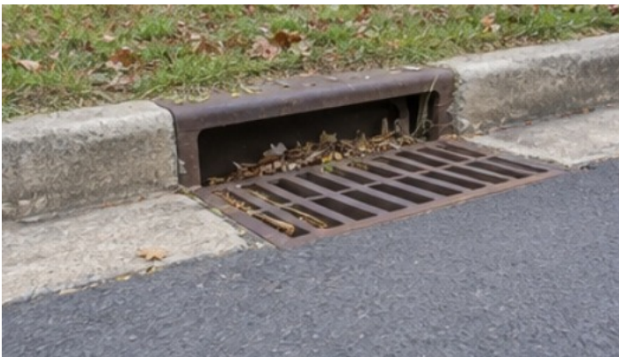
Photo 6: Catch basin at the curb.
