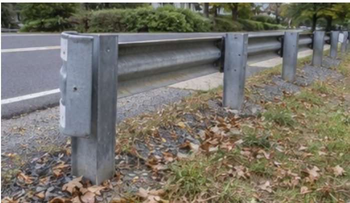
Photo 4: Roadside guardrail and support posts.
