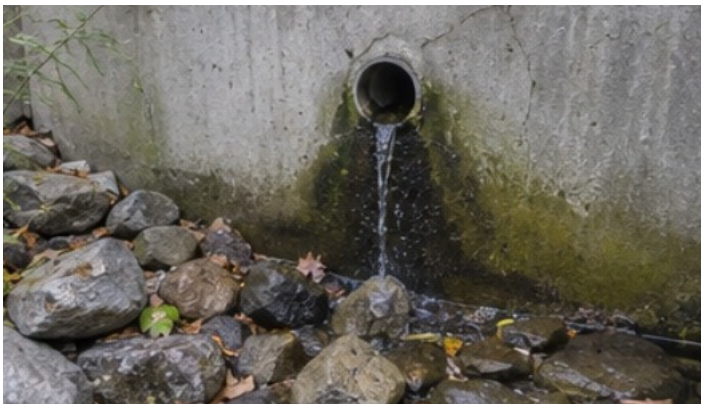
Photo 7: Retaining wall drainage outlet.
