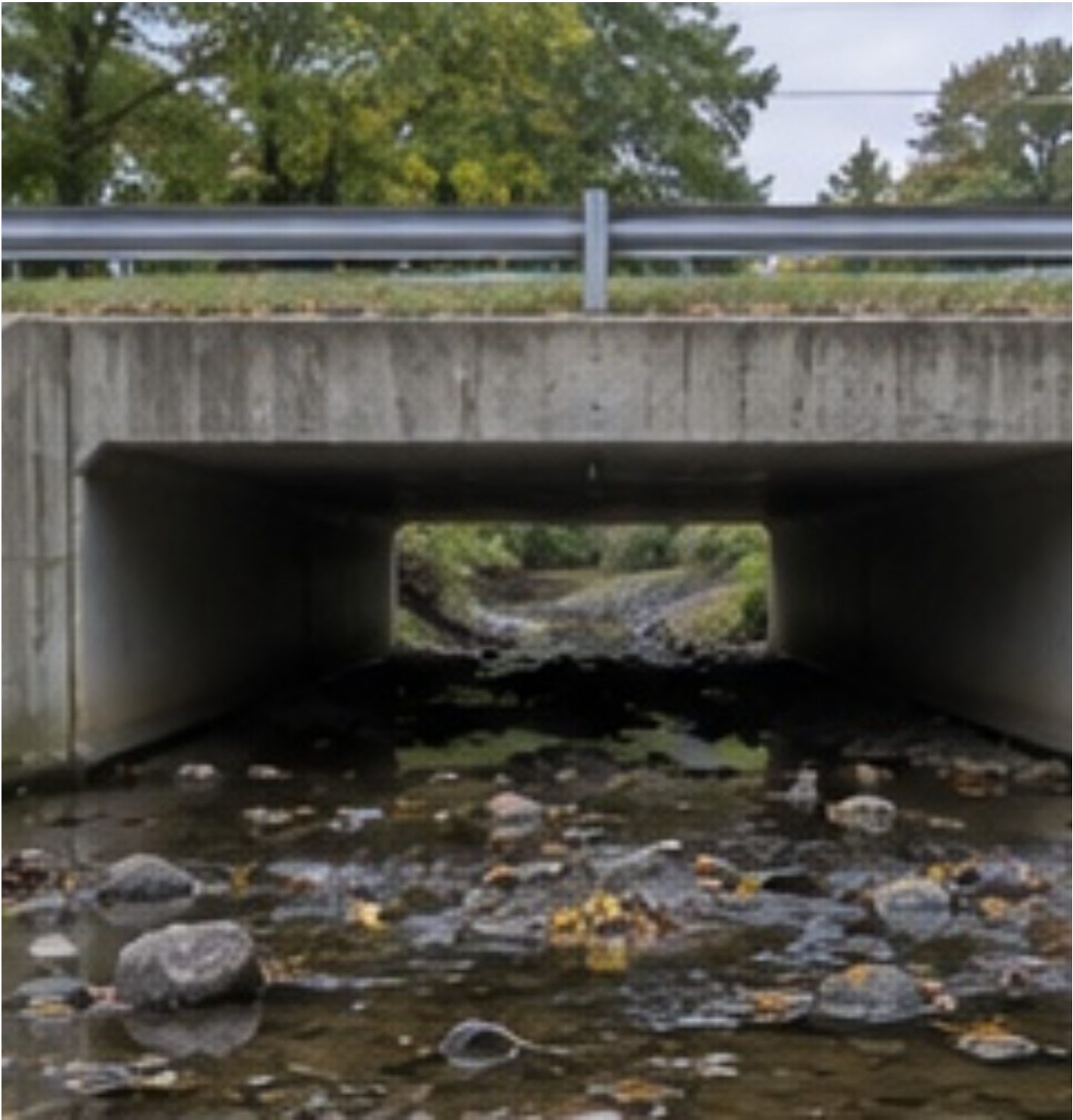
Photo 1: Culvert inlet and road embankment.
