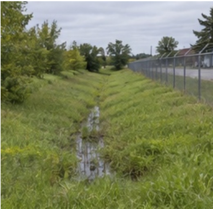
Photo 4: Surface drainage along the property boundary.
