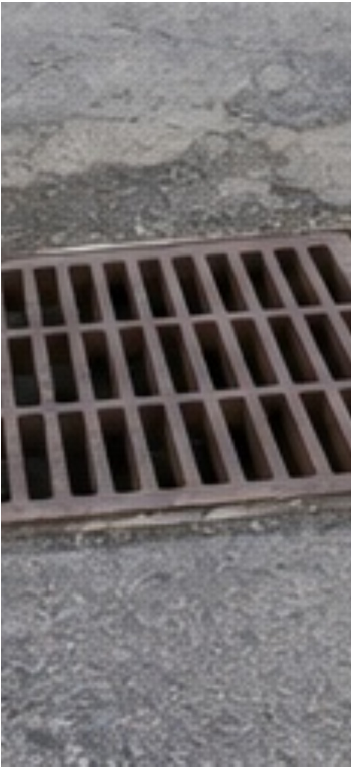
Photo 6: Catch basin in the paved service yard.
