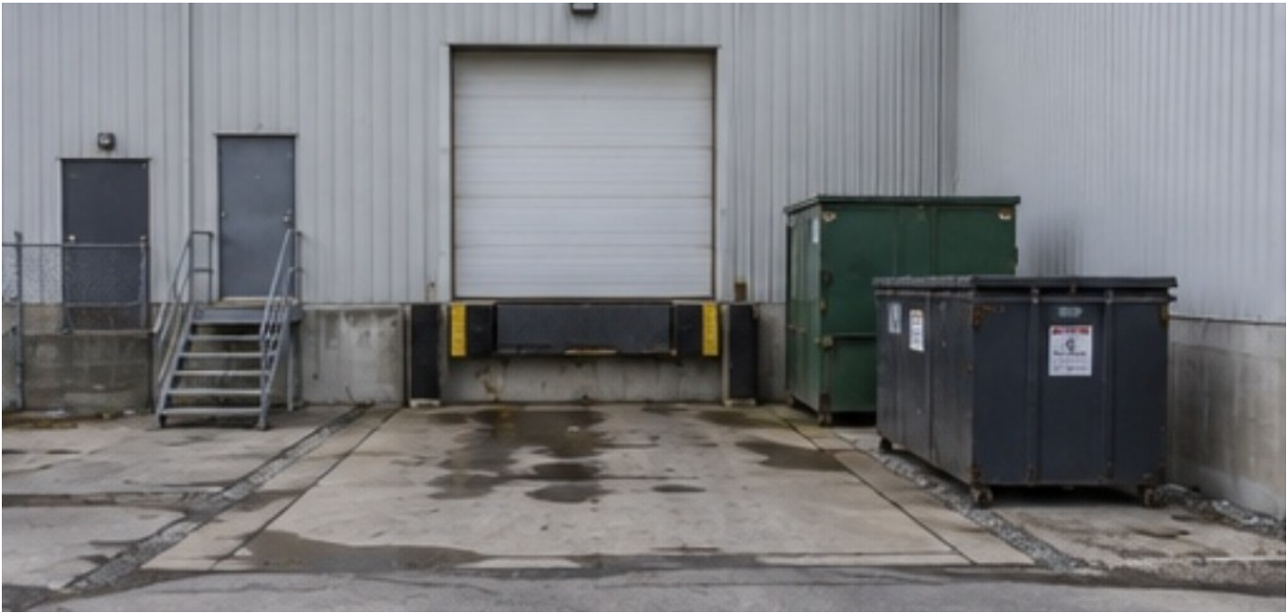
Photo 8: Loading dock and waste storage area.
