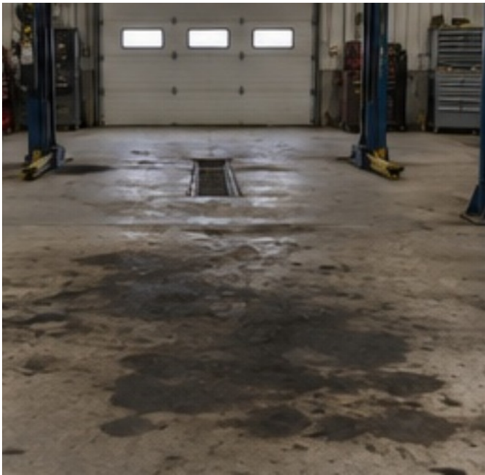
Photo 5: Concrete condition in the vehicle maintenance bay.
