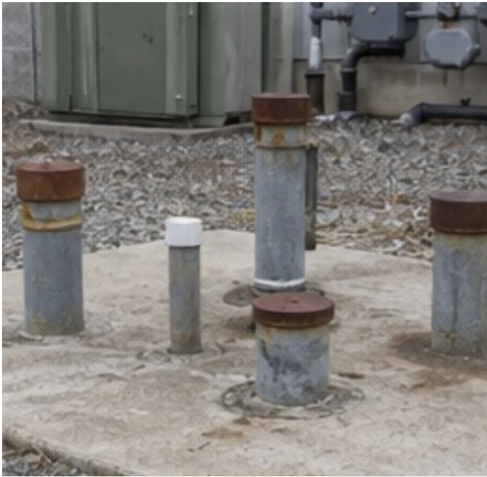
Photo 3: Capped service connections at the former equipment pad.
