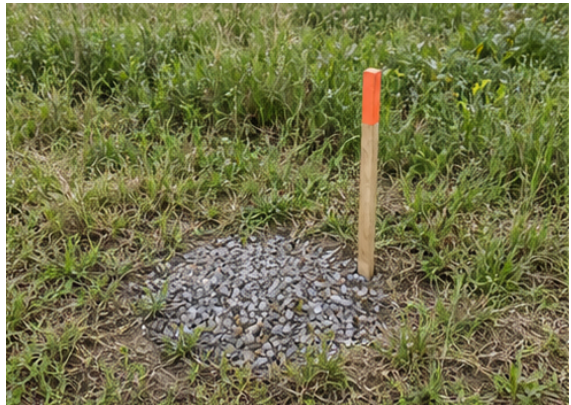
Photo 6: Completed borehole location following reinstatement.
