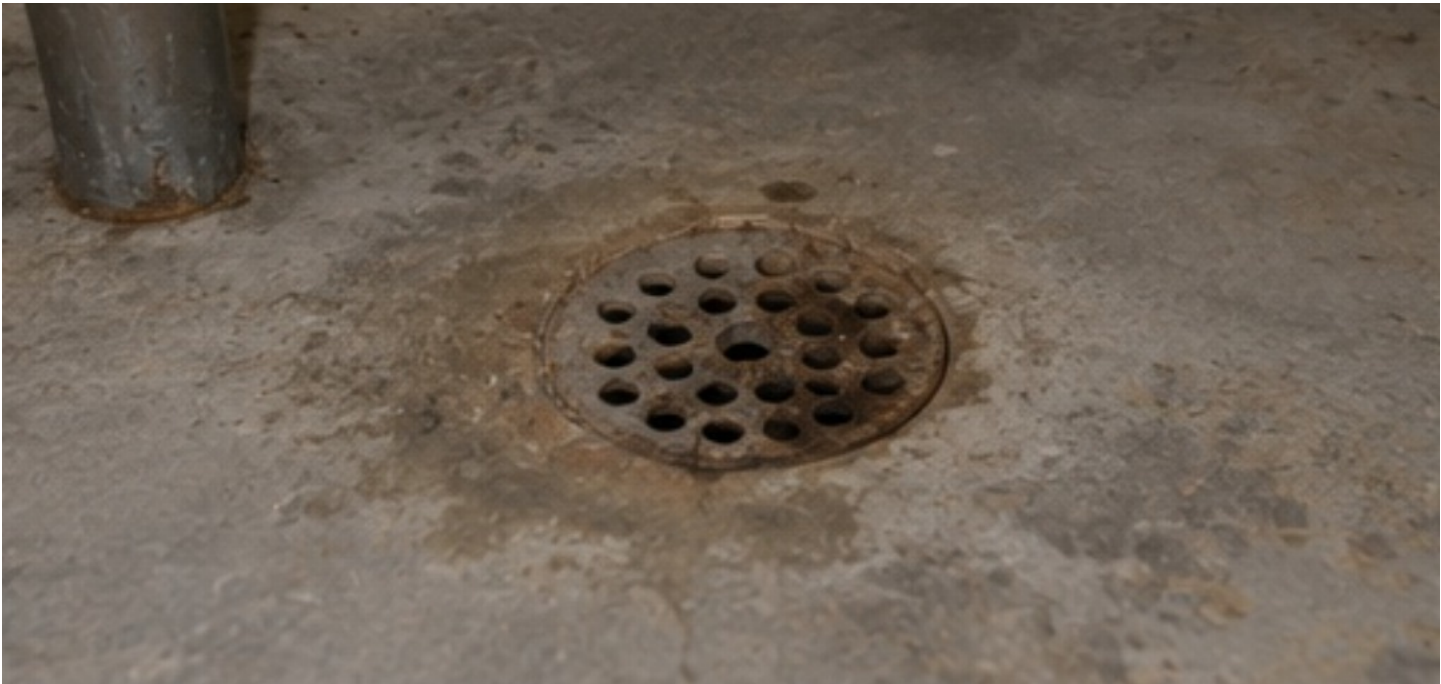
Photo 8: Basement floor drain.
