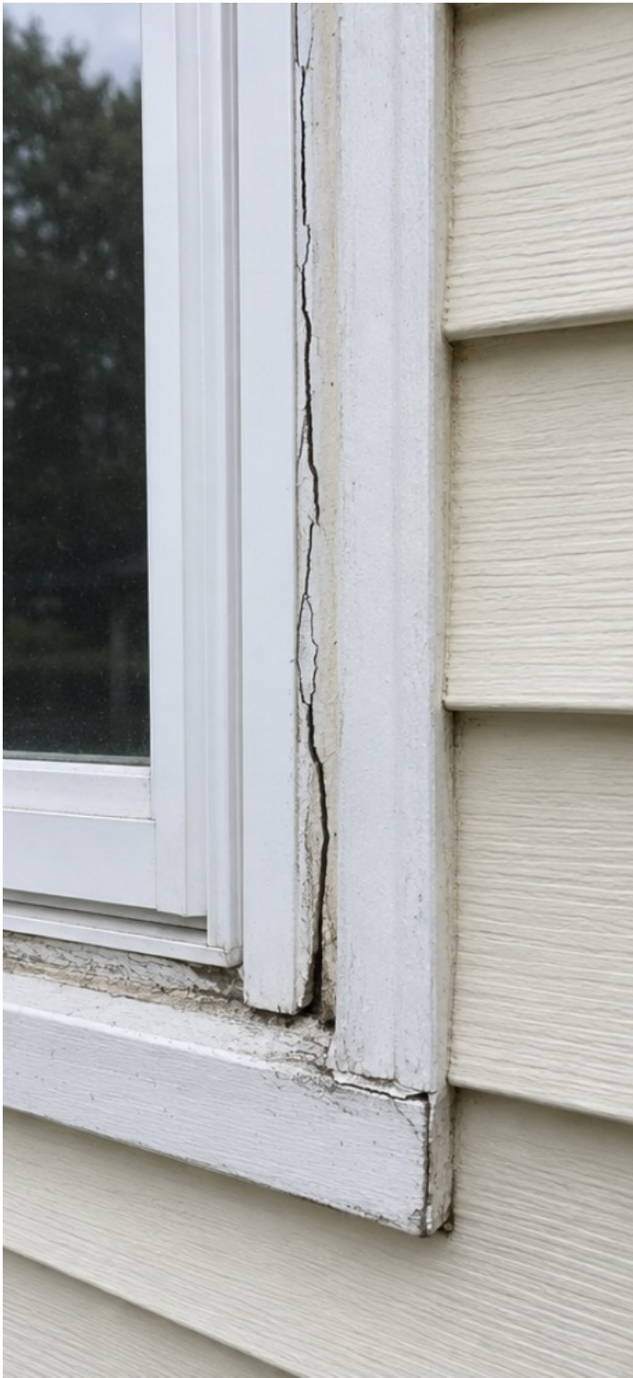
Photo 6: Window perimeter sealant condition.
