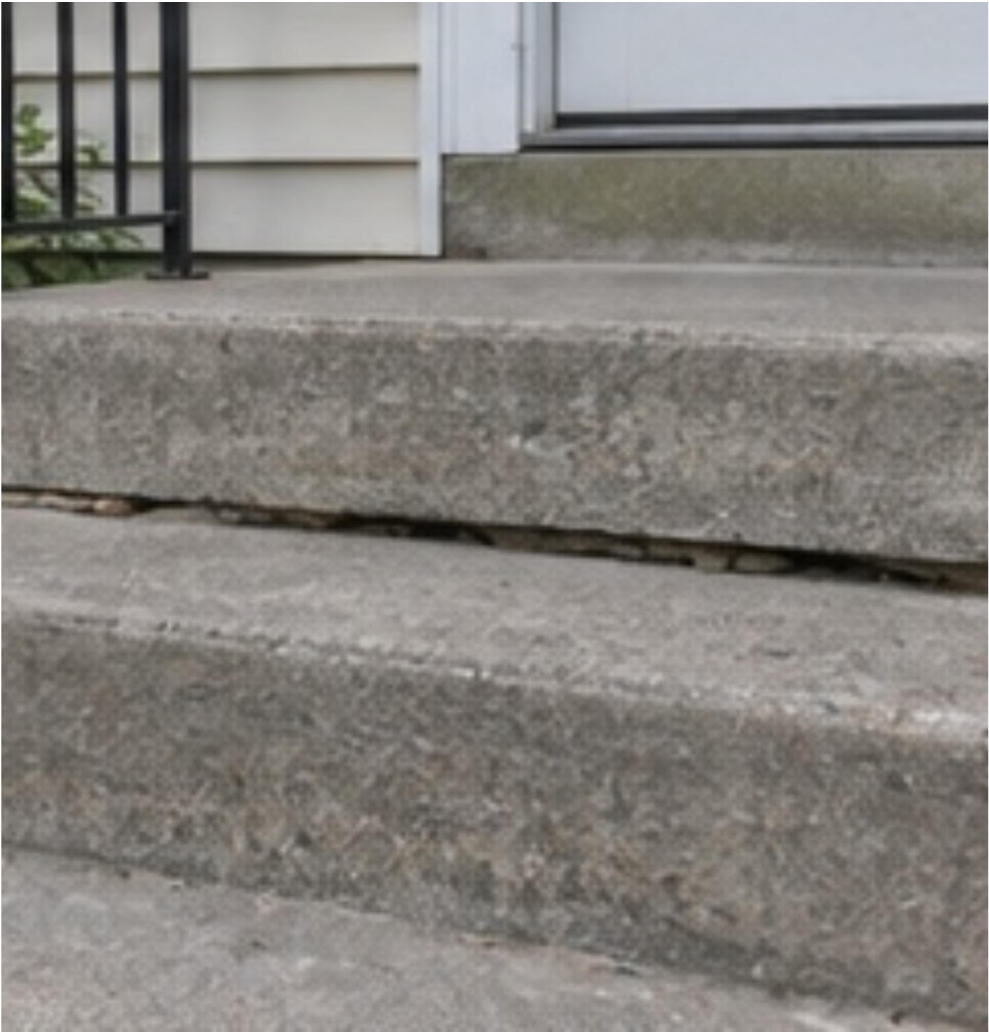
Photo 7: Concrete entry step condition.
