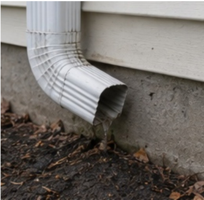
Photo 3: Downspout discharge beside the foundation.
