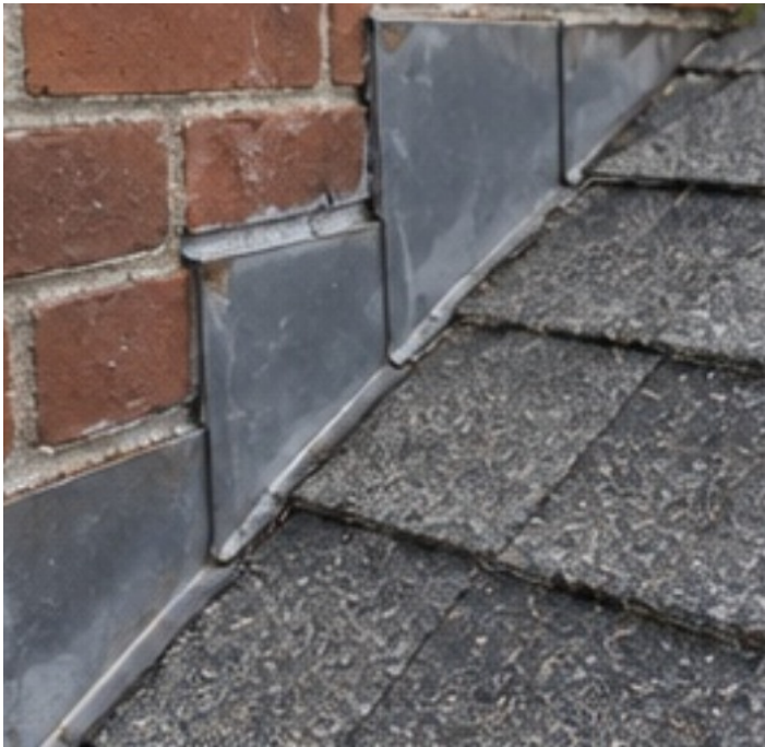
Photo 5: Step flashing at the chimney.
