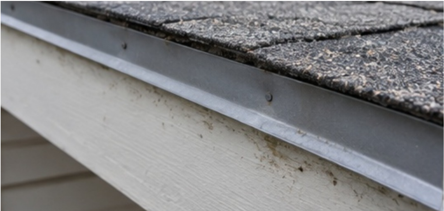
Photo 8: Drip edge and fascia detail.
