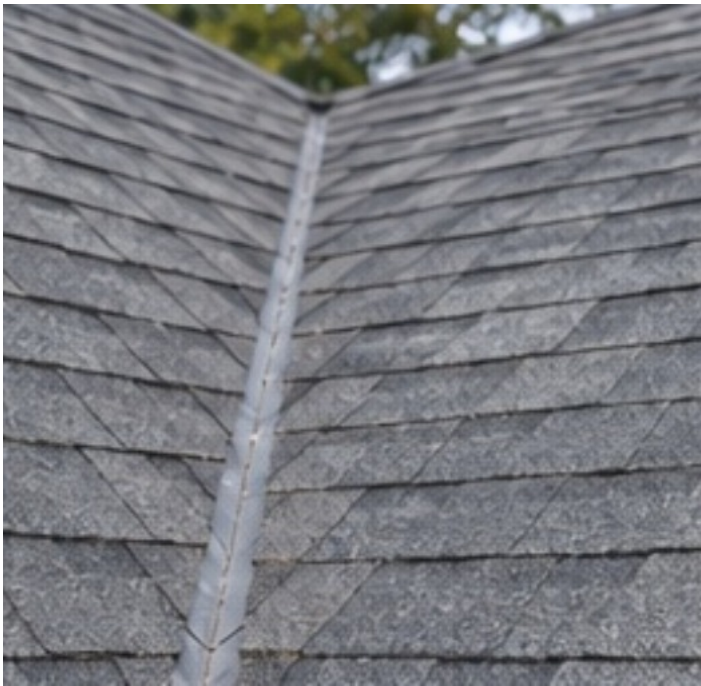
Photo 7: Roof valley and intersecting slopes.
