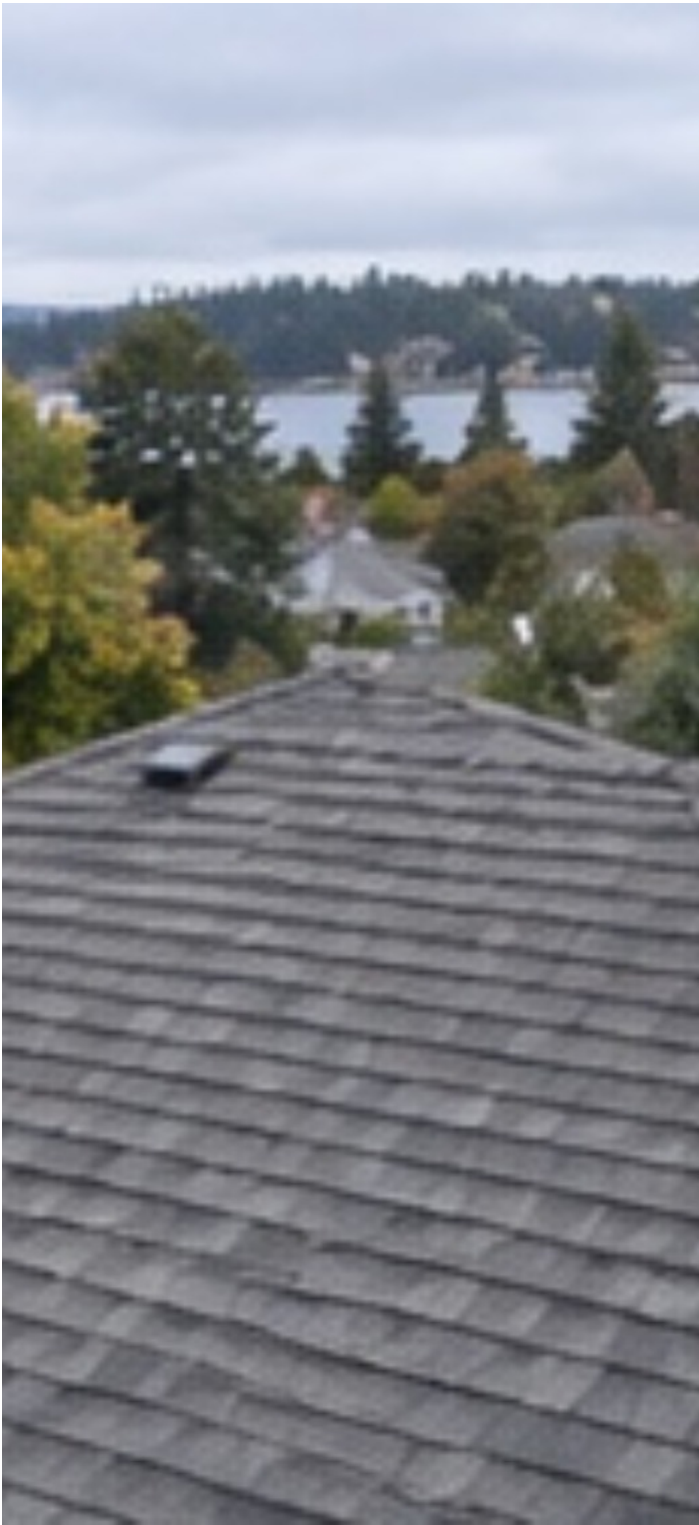
Photo 1: Overview of the roof and chimney.
